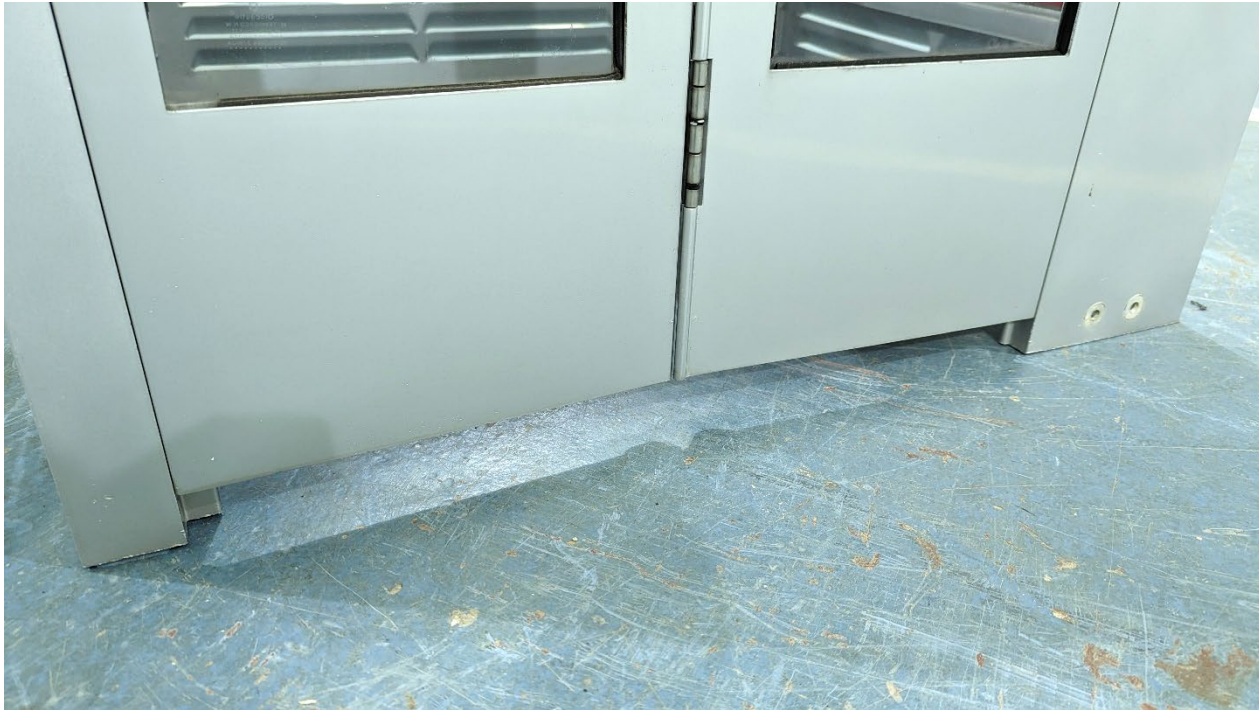
Figure 3 – Detail of gap underneath specimen door
