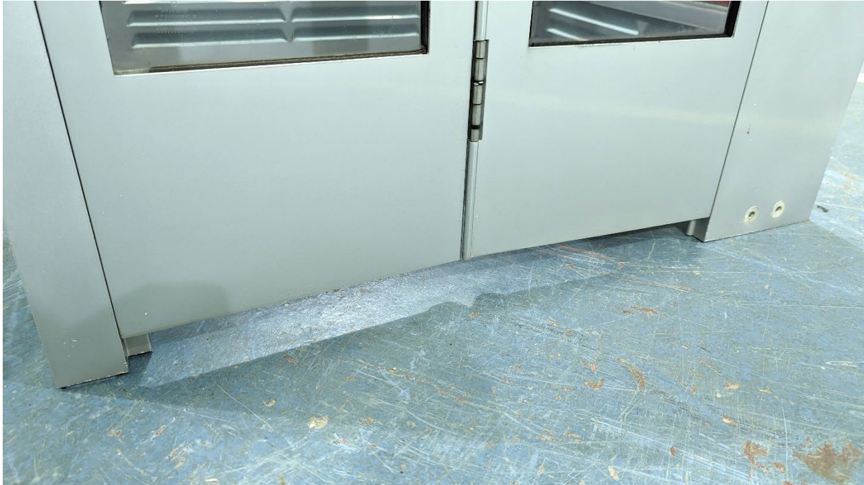
Figure 2 – Detail of gap underneath specimen door
